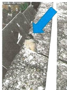
Broken parapet
