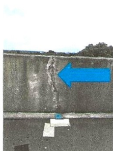
Roof walling cracked
