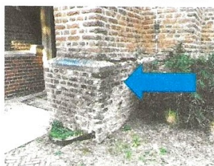
Broken parapet
